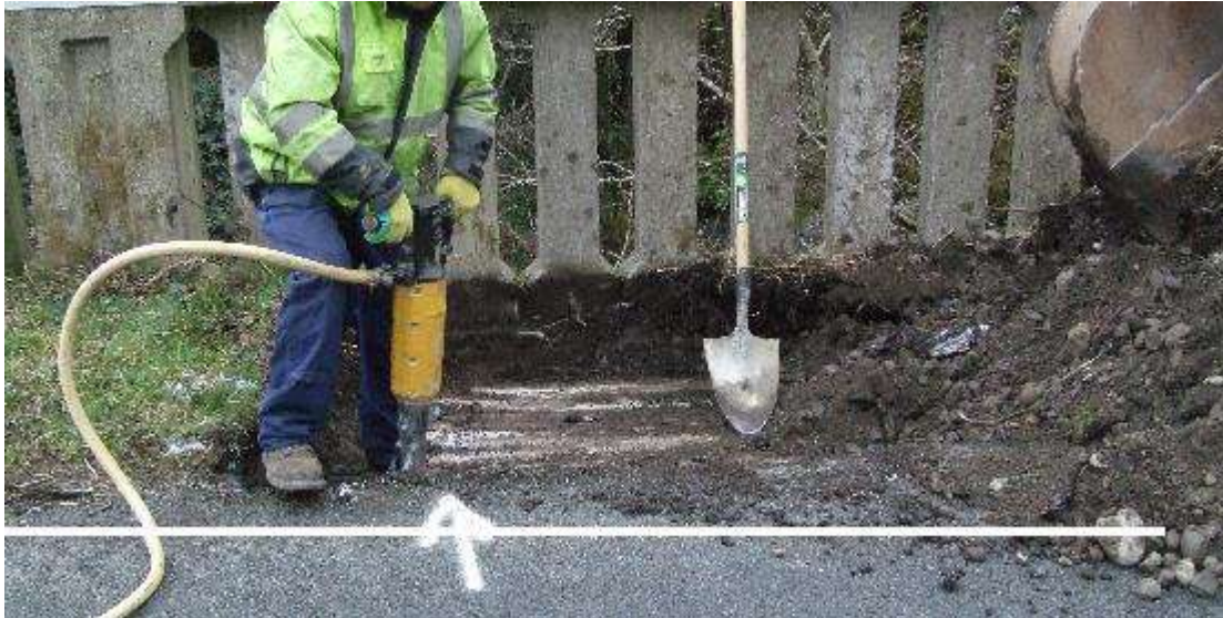
Excavation for structural assessment of Spearpoint Bridge, Ballymurphy
