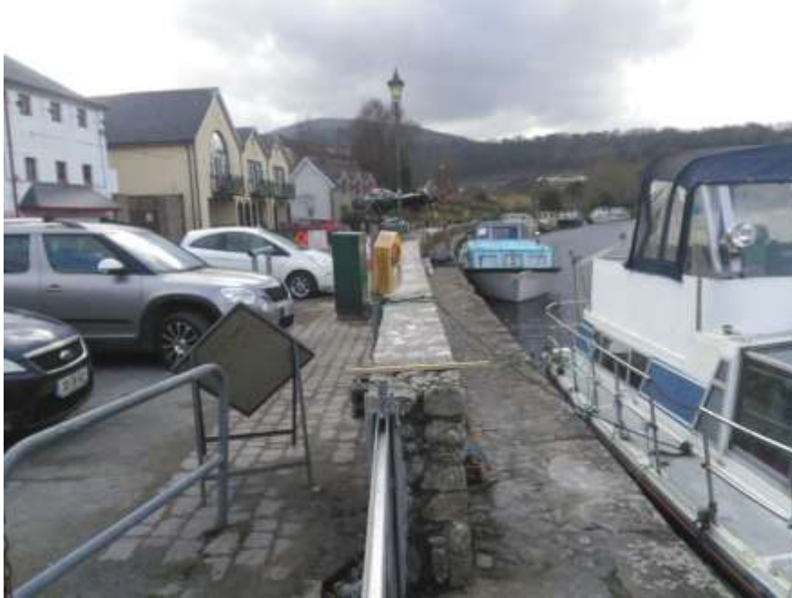
New wall at Tinnahinch
