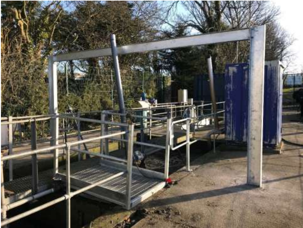
New Gantry & Walkway at Nurney WWTP
