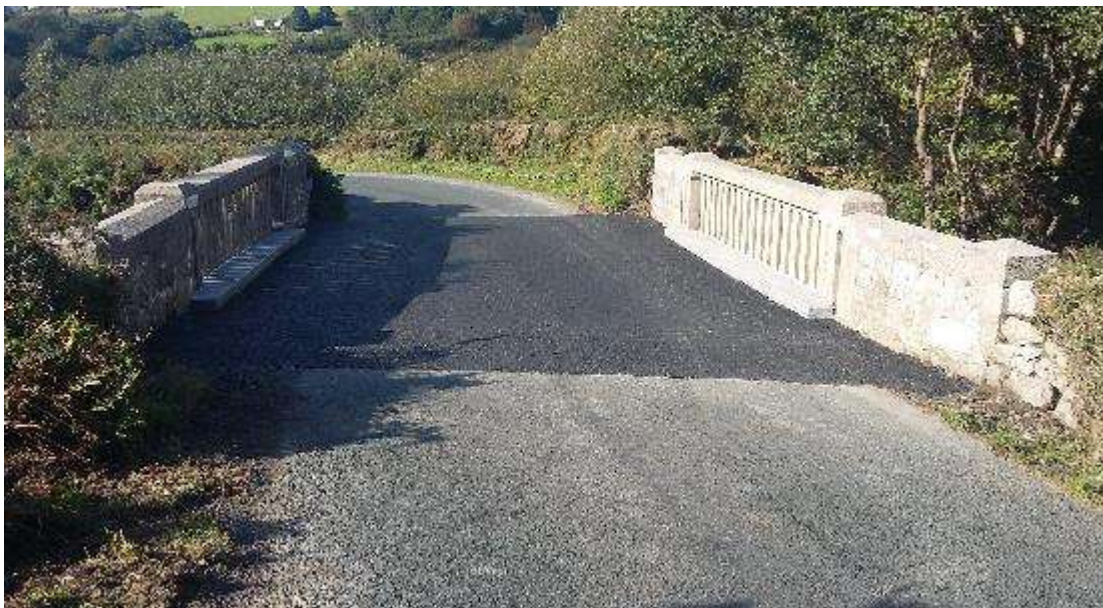
Completed Repairs to Spearpoint Bridge, Ballymurphy
