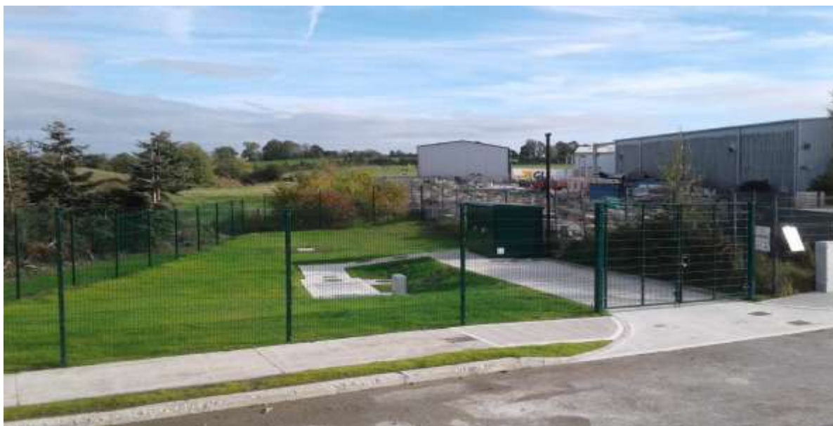
Wexford Road Pump Station
