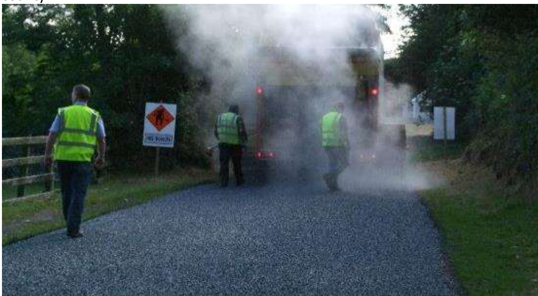
Restoration Maintenance Operations (Surface Dressing)
