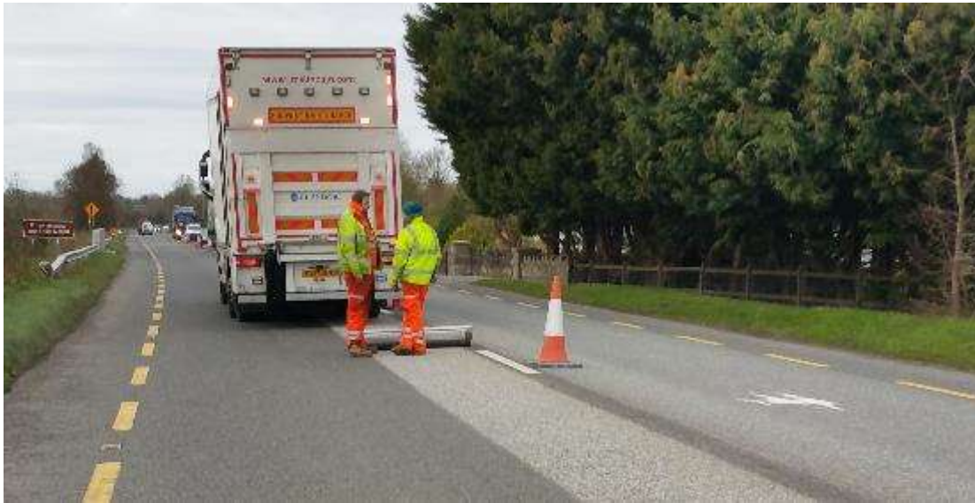
Re-texturing in progress on the N80
