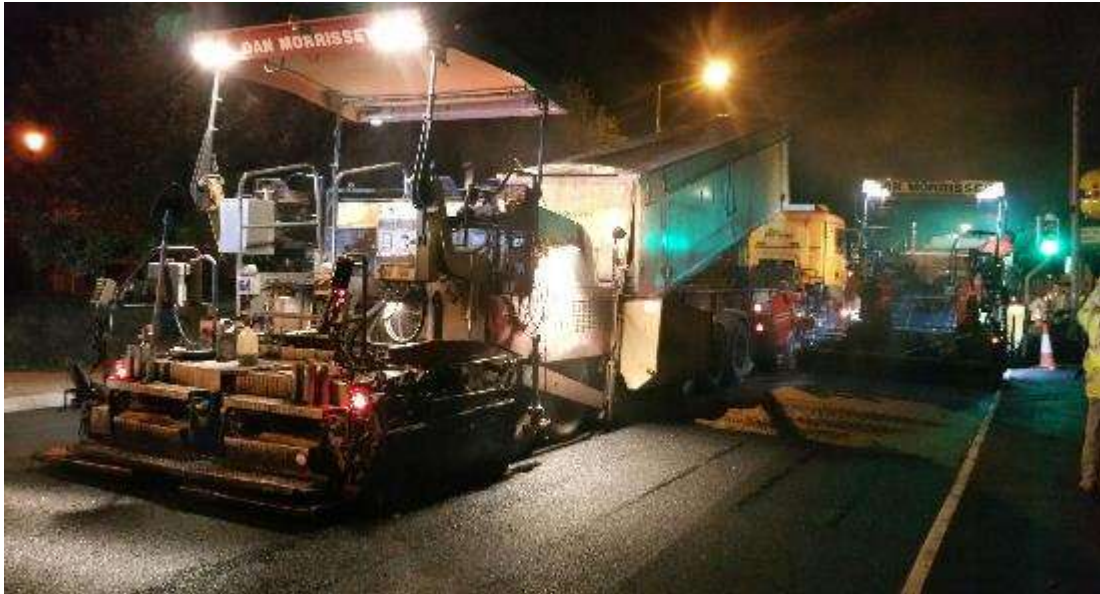
Night time works on the N80 project, Tullow Road, Carlow Town
